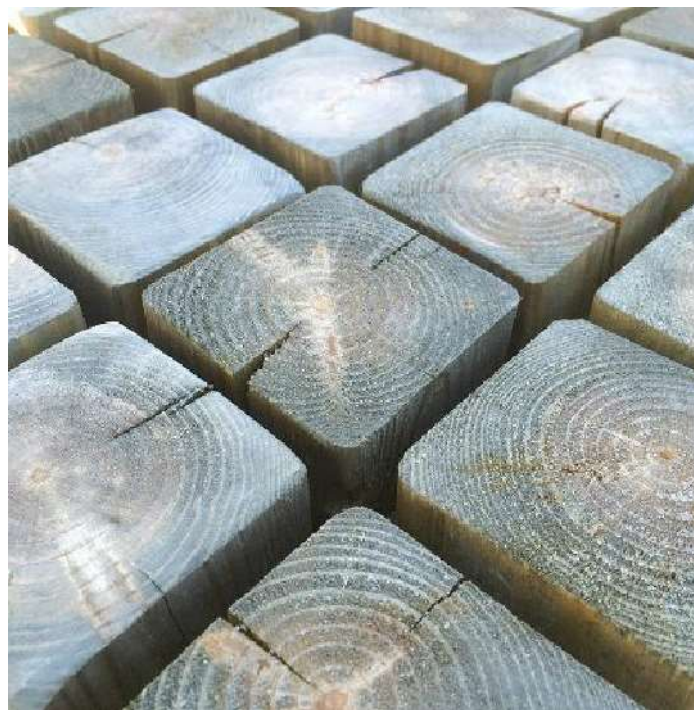
The path is made from reclaimed 4x4s.
